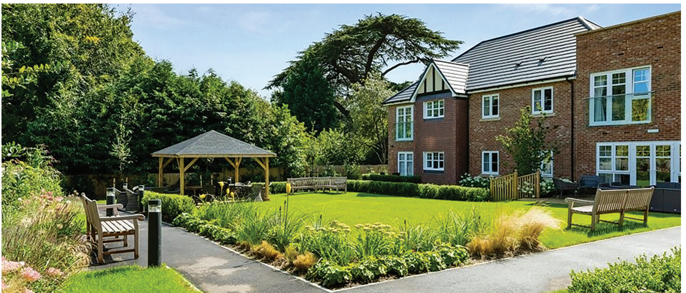
Existing scheme at Sanderstead
