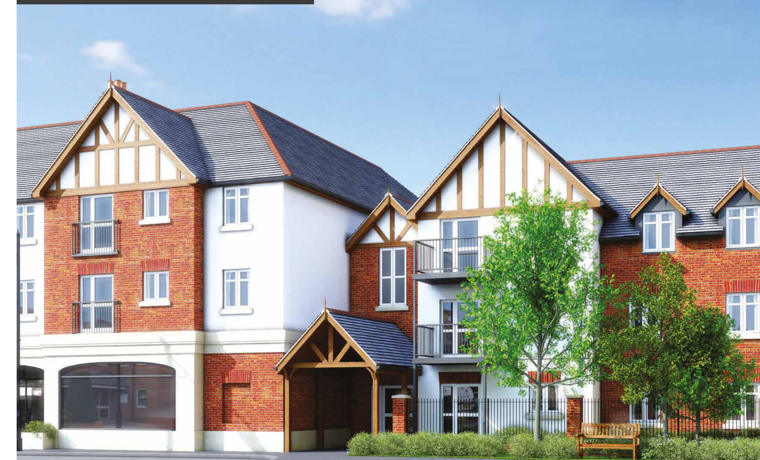
Existing development – Bourne End
