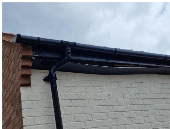
Plate 12. Soffit box with open access.
