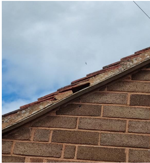
Plate 10. Mortar and roof tile gap.
