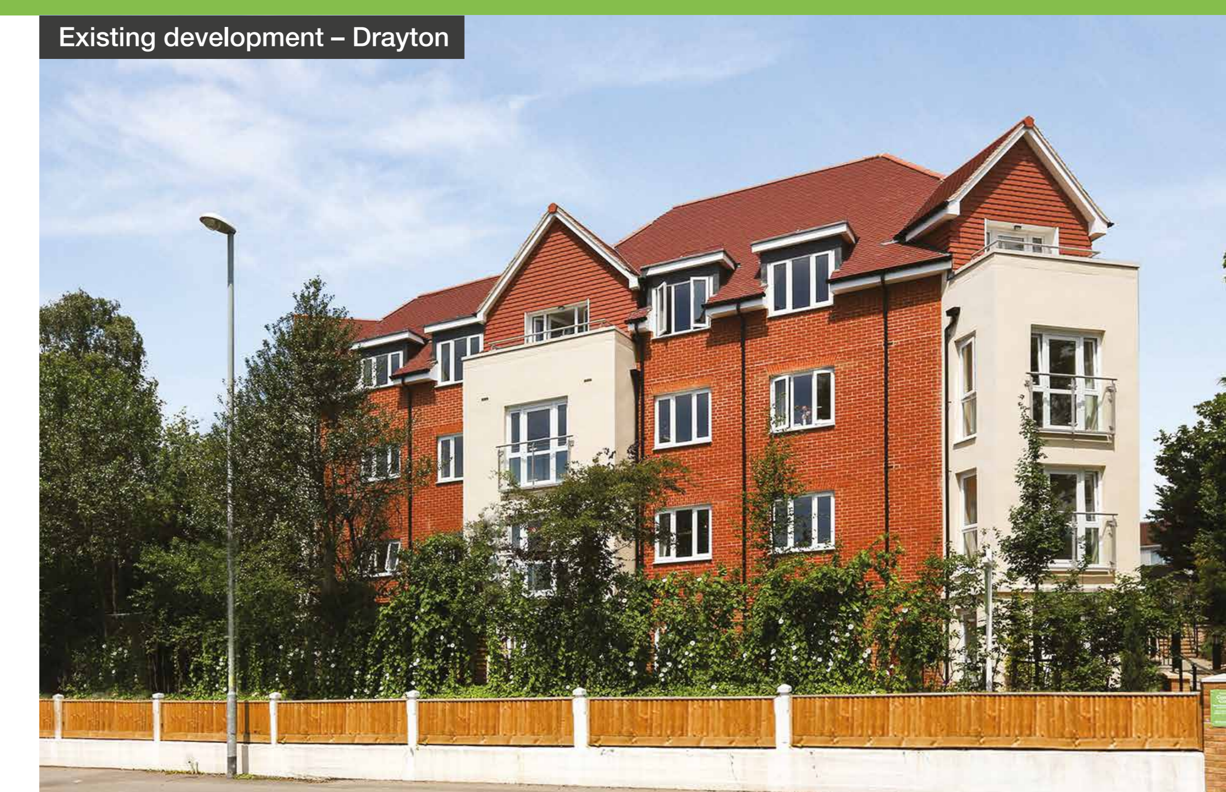
Existing development – Drayton
