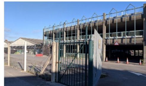
Existing multi-storey car park
