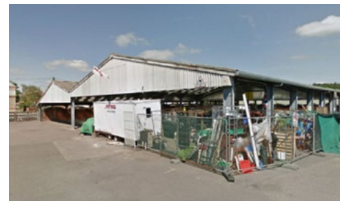
Existing market buildings
