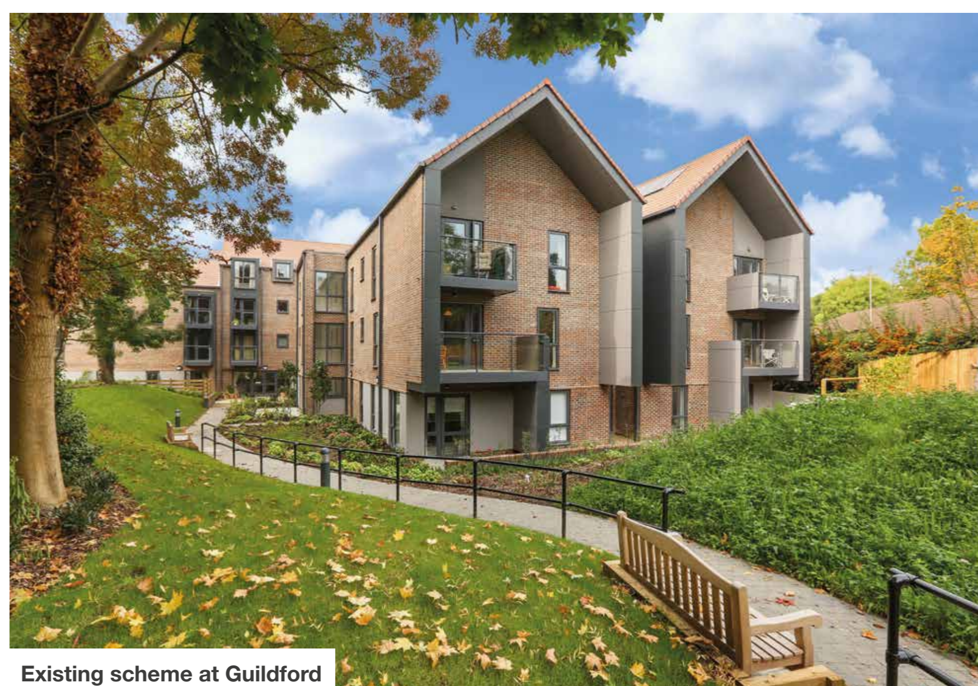
Existing scheme at Guildford
